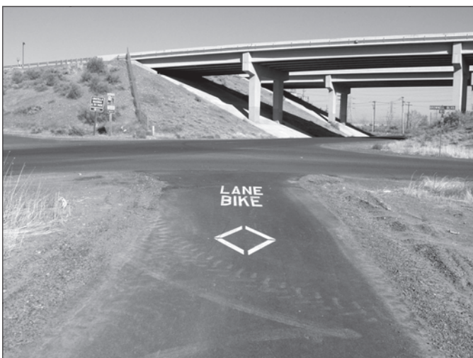
Path access on Brownell Blvd.
