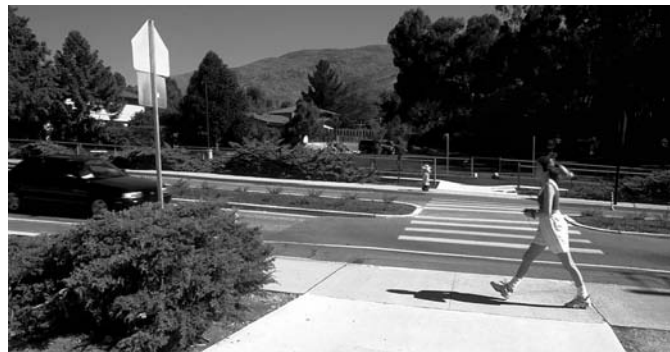
Refuge island with speed table and high-visibility crosswalk.
