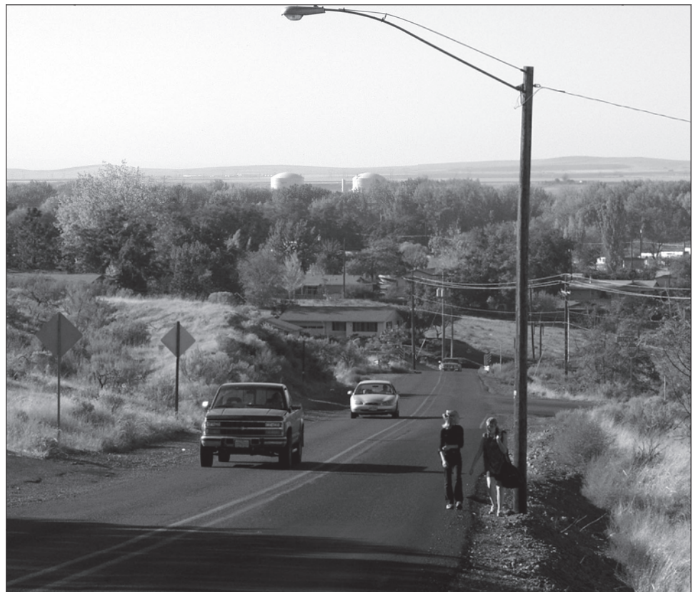
Powerline Road (north section) — primary access to South Hill has narrow, unpaved shoulders.
