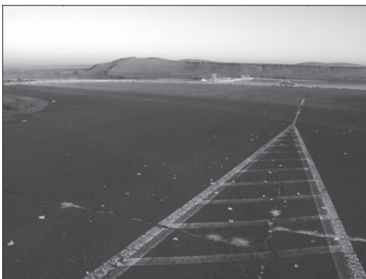
Large paved overlook could be made into an attractive stop near the Lewis & Clark Trail.
