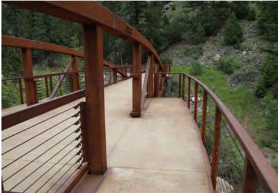
FIGURE 6 TRUSS WITH OUTBOARD PLATFORM
