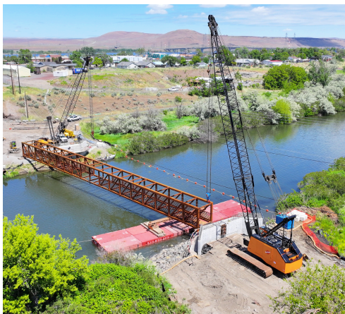
The Pedestrian Bridge atop abutments.
